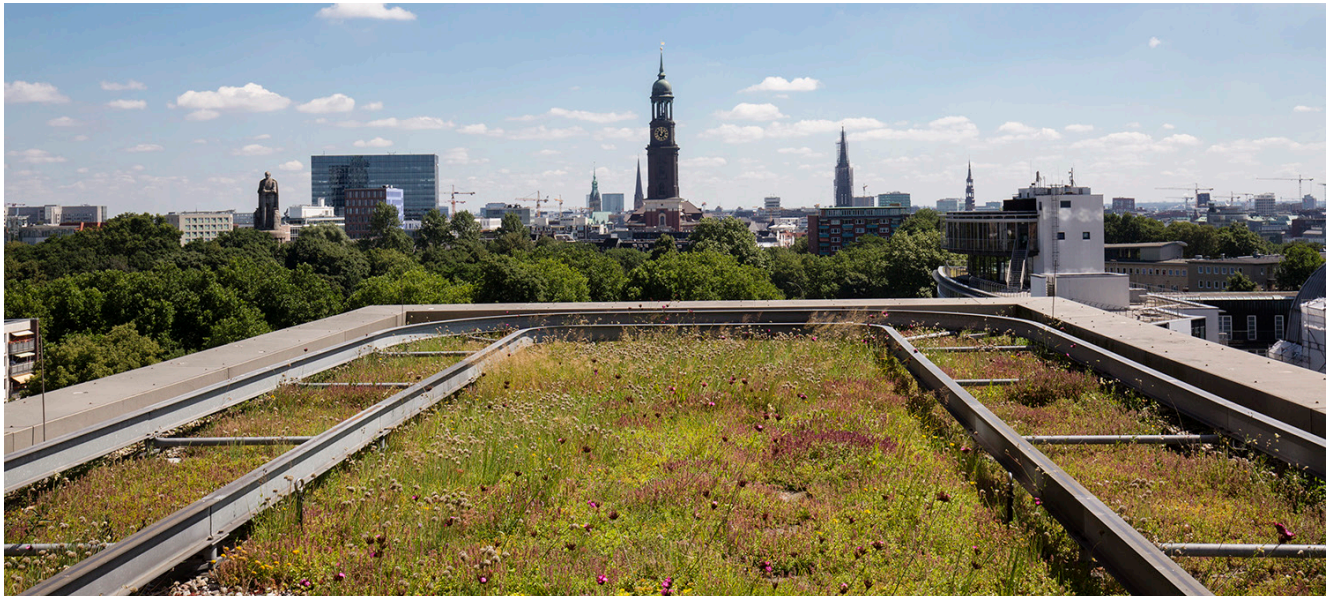
Green roofs can keep buildings cool during heat waves and insulate during cold winter months, decreasing energy costs. © BUE, Isadora Tast
